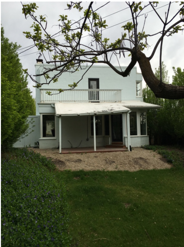
View of the rear of the property facing east
